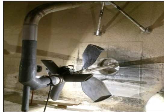
Mixer and lance with the applied ARC products
